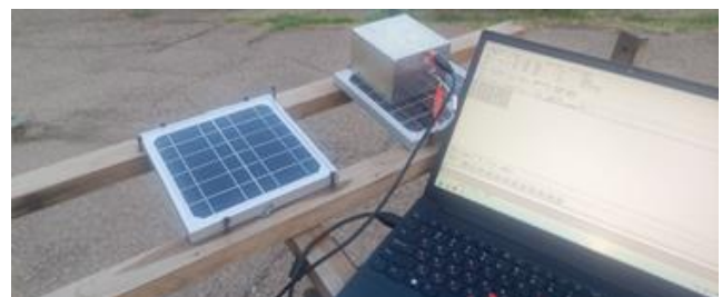
Fig. 2. Carrying out measurements by the device
